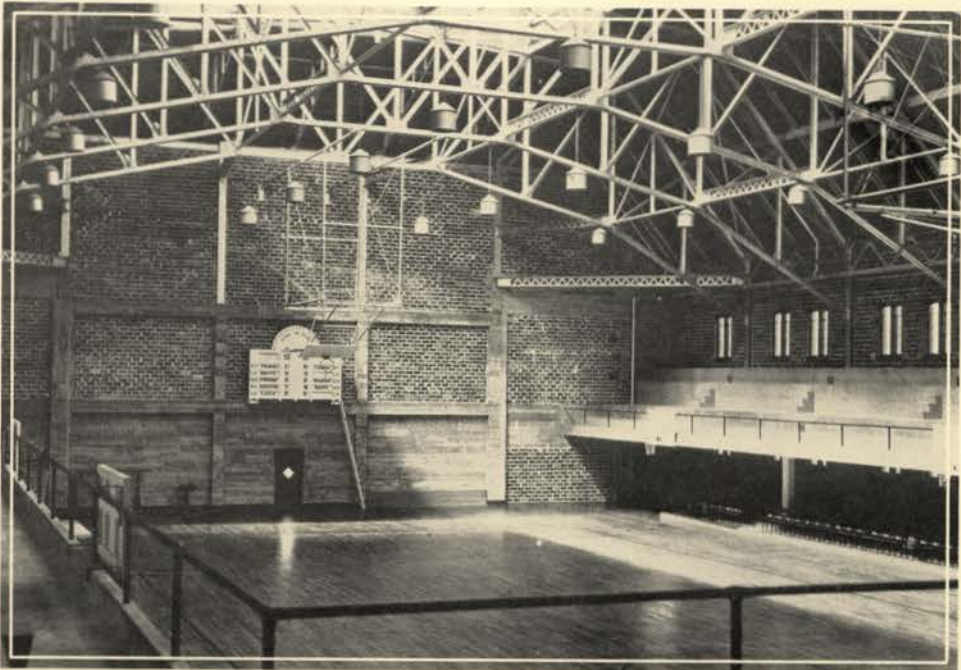
THE NEW FLOOR
