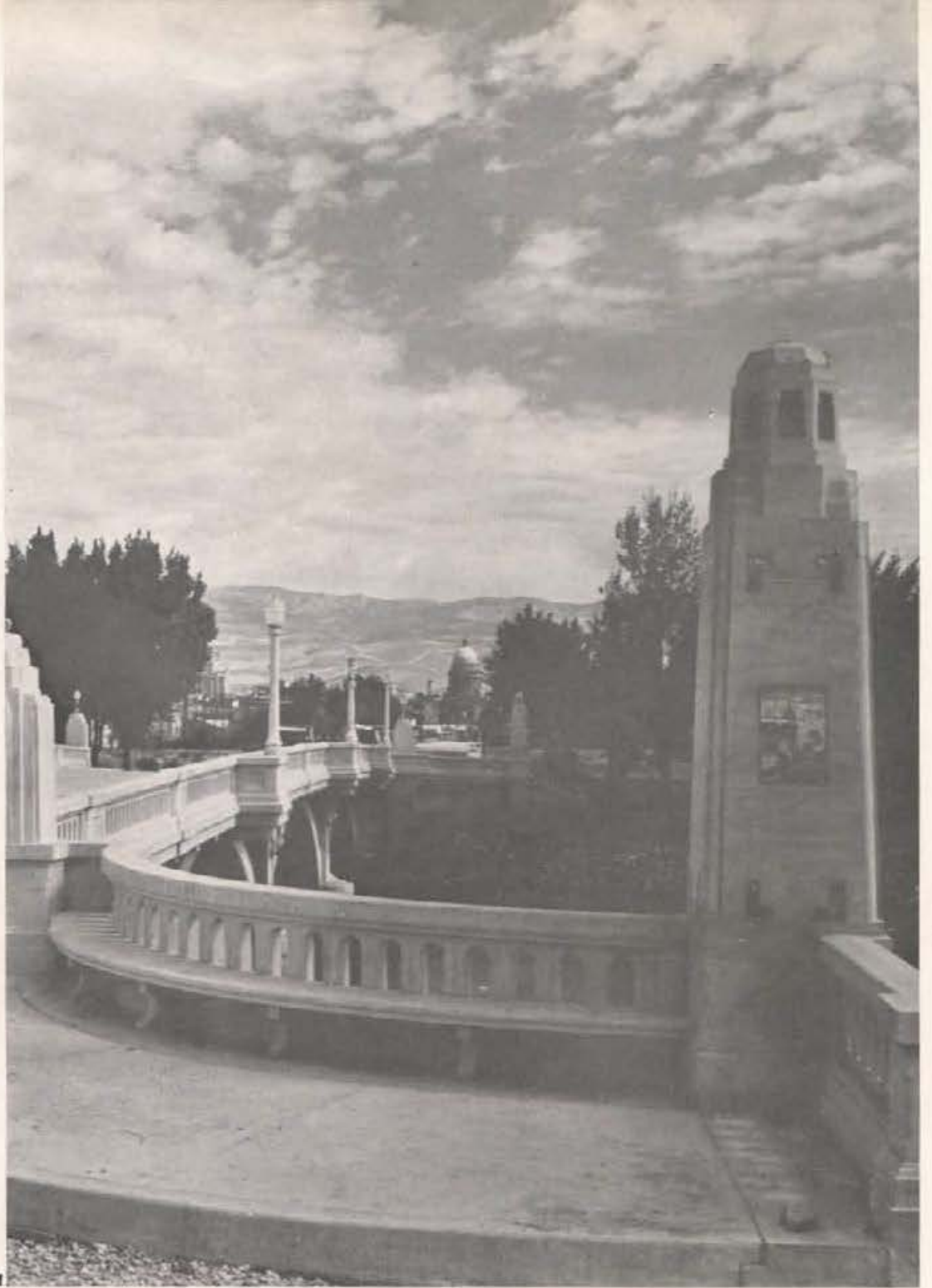
Looking down Capitol Boulevard: Oregon Trail Memorial Bridge—the Capitol in the distance.
