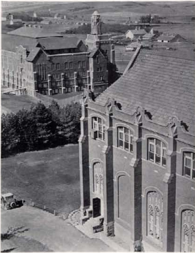
Back entrance to "Ad"
