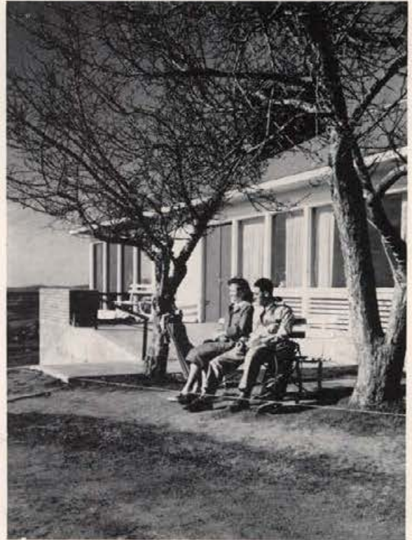
New ASUI-financed golf club house shortly after completion
