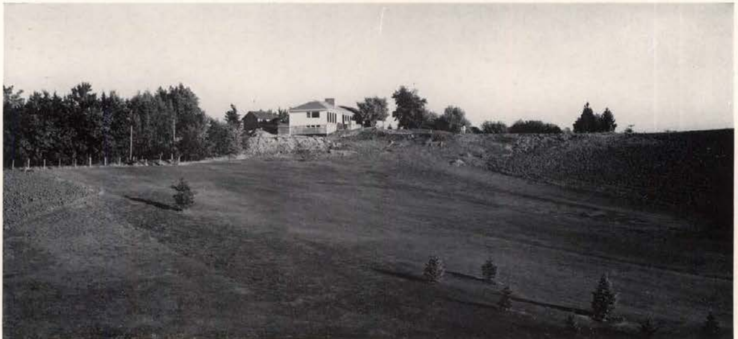
Situated on hill commanding a view of number one green and fairway, the golf club house was completed early in April
