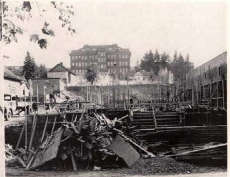
In the fall Kirtley Annex construction was just beginning.
