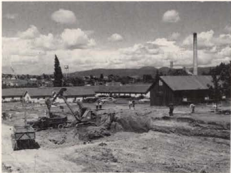
First excavation for the new Ag Science building was made June, 1949.
