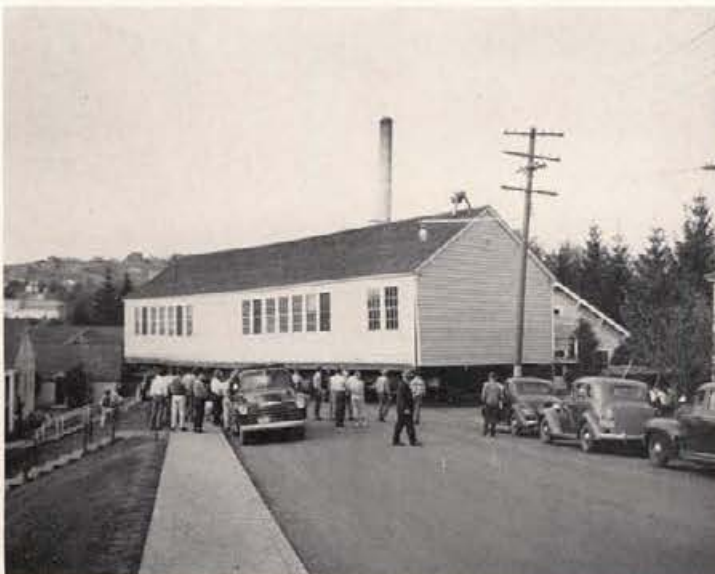
Three frame forestry buildings had to be moved to clear the space for the Engineering Classroom Building. Here the wood conversion laboratory is shown precariously turning a corner on the jaunt to its new home near Pine Hall.
