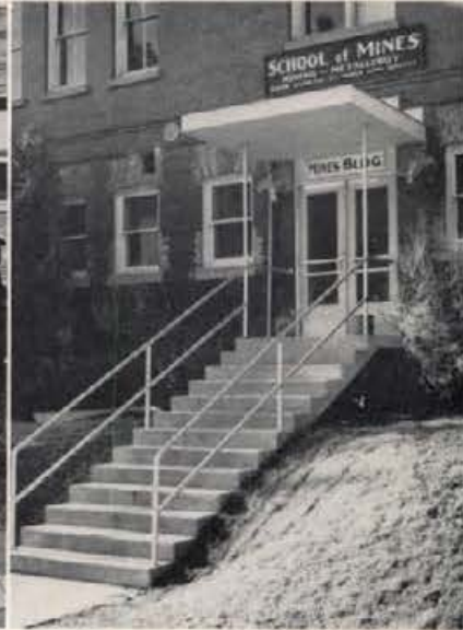
A new entrance-way dresses up the old School of Mines building which houses huge machinery employed in training future mining men for Idaho's vast mineral resources.
