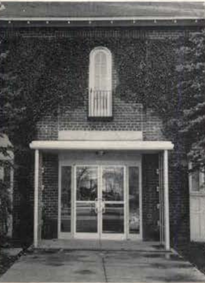
Hugging evergreens and an iron wrought balcony are two unchanged features of a newly-remodeled building.
