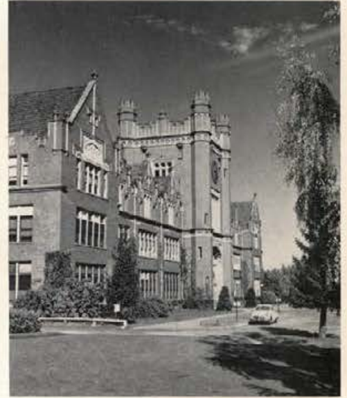
Familiar to every Idahoan's heart is the picturesque Administration building facade surveying the lawn and circular drive.
