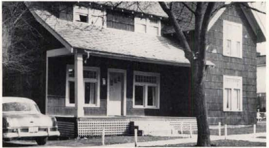
Chapter House at 730 Deakin Street
