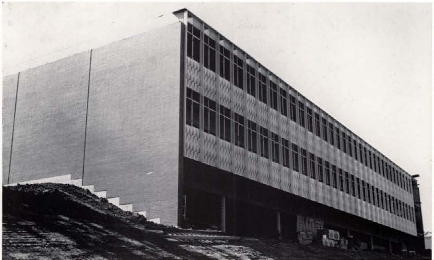
Above is the nearly completed Mines Building. The three-story, 190-foot structure costing $500,000 will be completed in September, 1961
