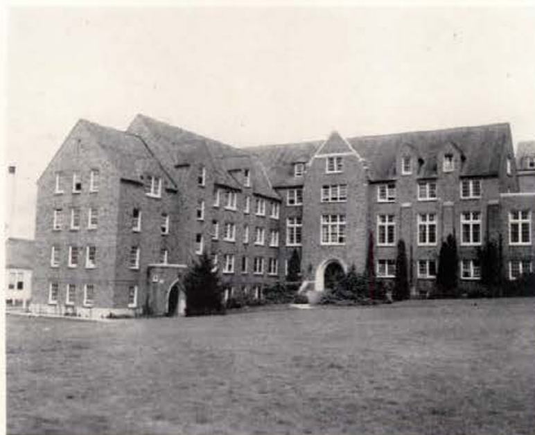
Chrisman Hall Idaho Avenue
