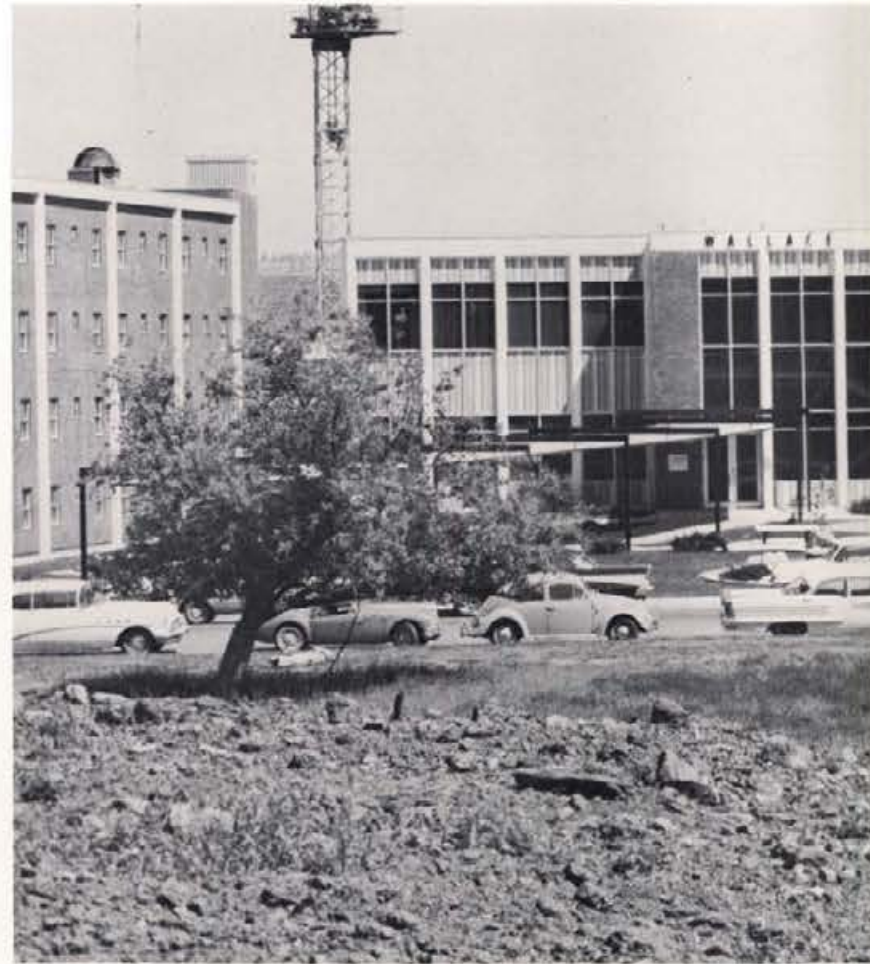
The Wallace Complex, composed of Campbell, Carter, and Houston Halls for women and Borah, Graham, Lindley, and Snow Halls for men, currently houses 784 U. of I. students. The completion of fourth wing, now under construction, will add three halls and 336 students to this total. The complex also includes a large kitchen, several dining halls and lounges, and the offices of student and family housing.
