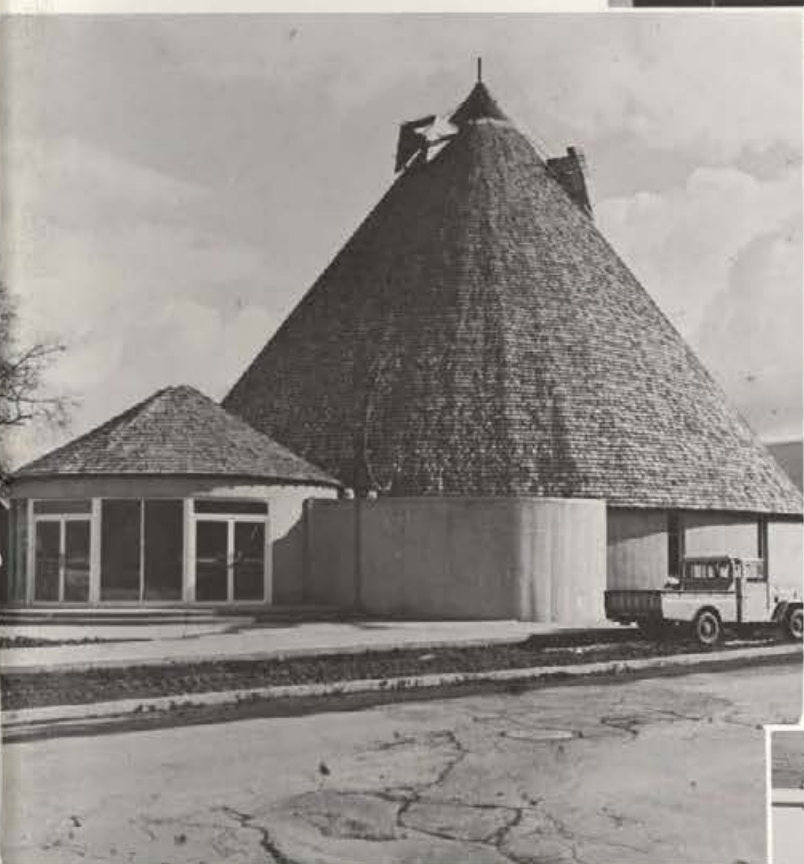
The New Catholic center on campus, St. Augustine's Catholic Center, was completed this year. The building contains a chapel with a seating capacity of 430, a chaplain's quarters, two classrooms, and a large meeting room. The official blessing dedication was conducted on May 7 with Bishop Sylvester Teimen of Boise leading the ceremony.
