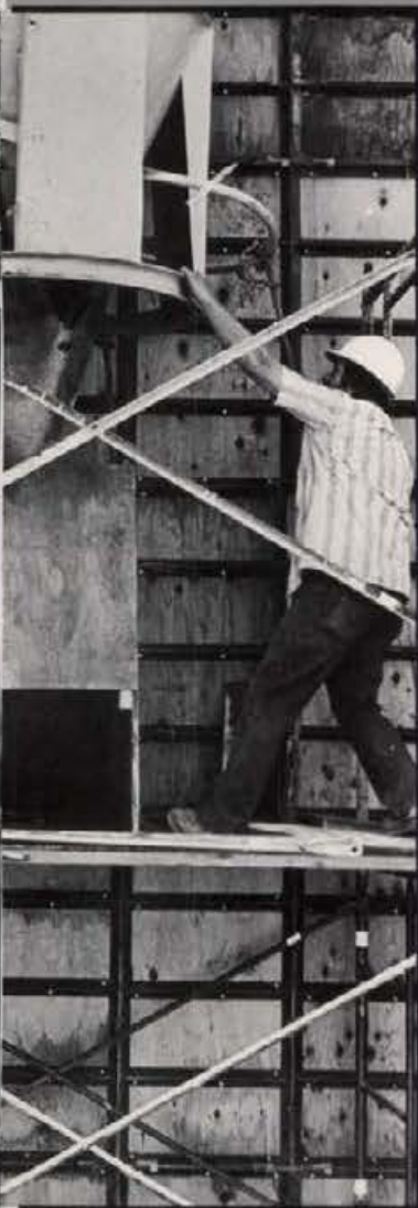
TWO CONSTRUCTION WORKERS balance precariously on the metal bracement as the cement flows into the walls of the East End Addition.
