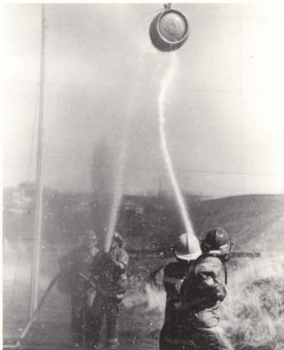
VOLUNTEER FIREFIGHTERS practice using the fire hoses by pushing an empty keg back and forth on a wire. (Gadsby)
