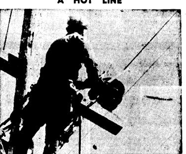
of the Washington Water Power Company, when emergencies arise. This man is shown working such a line in the territory where an insulator is to be replaced without an interruption in service. The picture was taken from "A Story of Electric Service."
