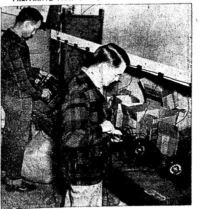
Walter Hilgert, shop repairman, left, and Mark Pederson, automatic switchman, Moscow, employees of the Interstate Telephone Co. testing phone sets for proper frequencies and ringing before equipment for the new automatic dial system was installed at Genesee by the company Wednesday. The two men checked and adjusted 375 automatic phones, attached numbers and packed them for delivery to homes and places of business. ment for the new automatic dial system was installed at Genesee by
