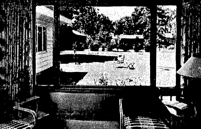
This window unit of ponderosa pine is ideal as a "picture" window. Fixed sash in center offers unobstructed view, casement sash on each side open for ventilation.
