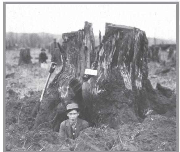
A lantern slide from Charles Houston Shattuck's classroom collection illustrating a method for stump removal. The caption reads: "Stump in Fig. 19 after blast. Charge was too small."
