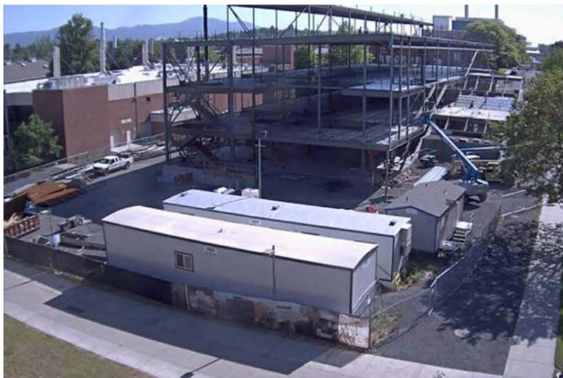
For the Integrated Research Innovation Center building (IRIC), our crew has completed the metal deck and is now moving into the next phase of construction. All concrete decks should be complete by the end of August. Hopefully we will be able to pour and dry the concrete before cooler weather closes in.
