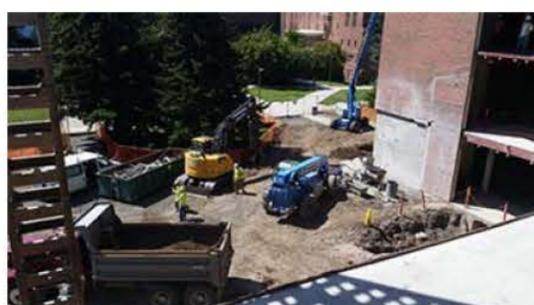
The College of Education building is also ongoing. Floor one is undergoing a rebar installation and doweling is in process in the sewer/waste line
