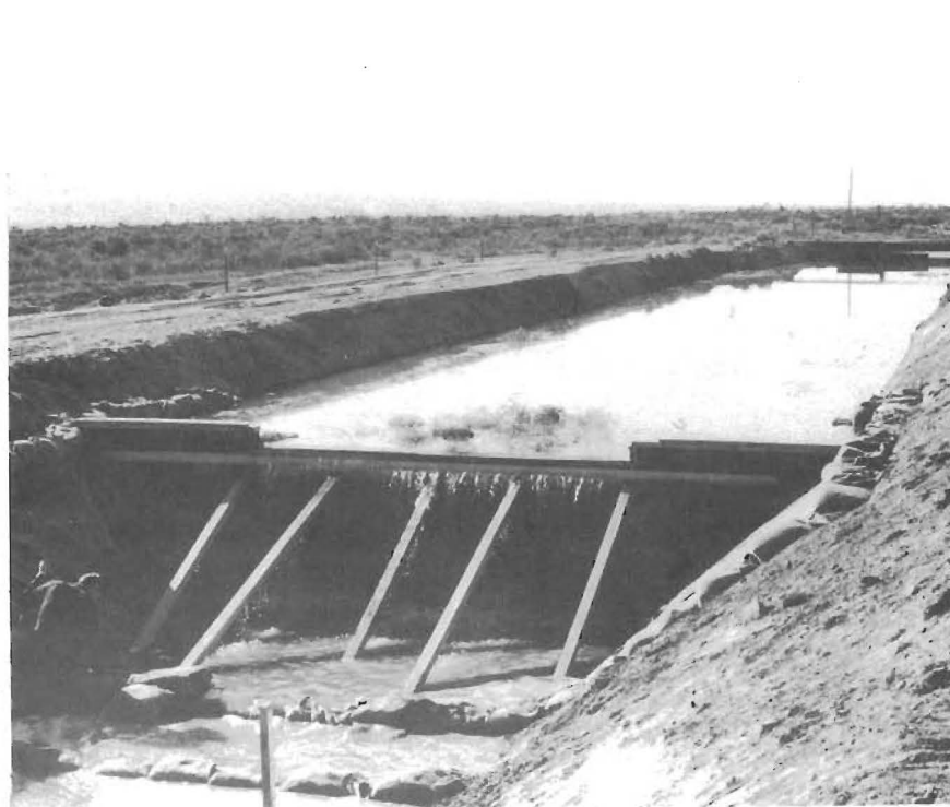
A. Construction of plywood panel bulkhead, looking upstream.
