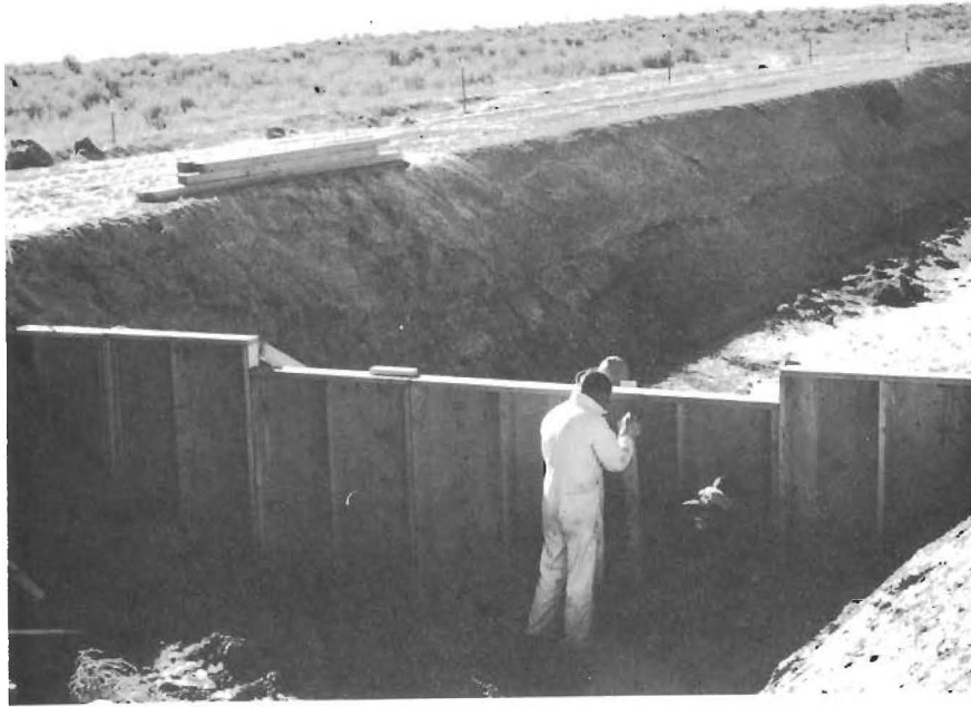
A. Construction of plywood panel bulkhead, looking upstream.
