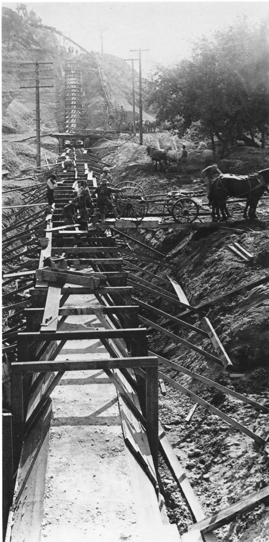
Repairing the break in the New York Canal.
