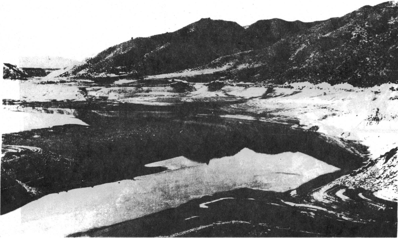
Figure 10. Looking Upstream from the North Bank of the Boise River, Arrowrock Dam, September 6, 1940.
