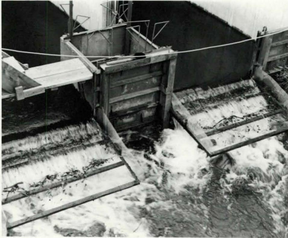
Figure 14. Upstream weir and trapping structures used during the spring and summer 1979 reduced stream discharge experiments, Troy Instream Flow Research Facilities, Grande Ronde River, Wallowa County, Oregon.
