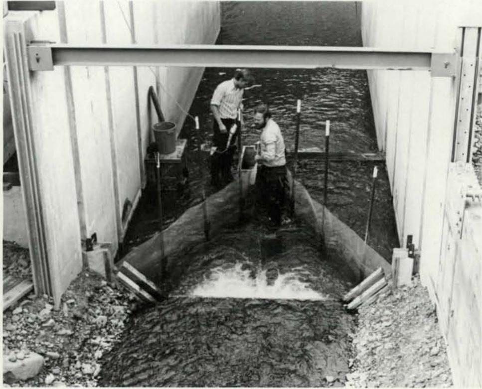
Figure 11. Downstream weir and trapping structures of the Troy Instream Flow Research Facilities, Grande Ronde River, Wallowa County, Oregon.
