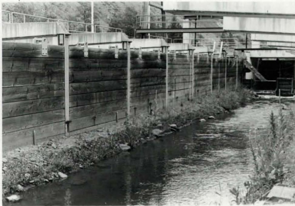
Figure 9. Simulated stream channel of the Troy Instream Flow Research Facilities, Grande Ronde River, Wallowa County, Oregon. Upper photo depicts the west channel at approximately  $0.03 \text{ m}^3/\text{s}$  ( $1 \text{ ft}^3/\text{s}$ ) prior to vegetative growth. Lower photo depicts the west channel at approximately  $0.28 \text{ m}^3/\text{s}$  ( $10 \text{ ft}^3/\text{s}$ ) after vegetative growth.
