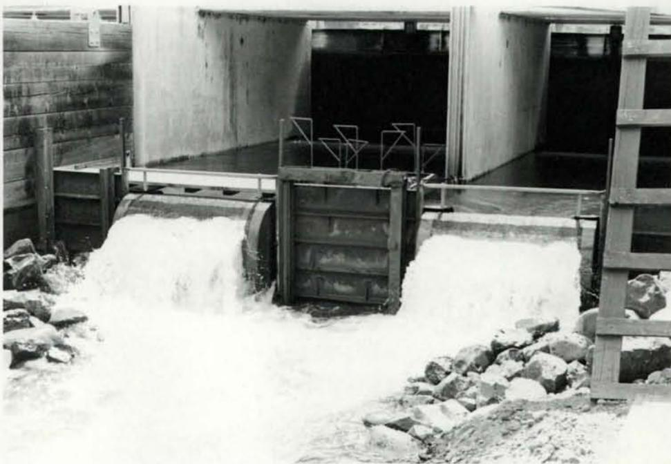
Figure 10. Upstream weir and trapping structures used during the fall 1978 reduced stream discharge experiment, Troy Instream Flow Research Facilities, Grande Ronde River, Wallowa County, Oregon.
