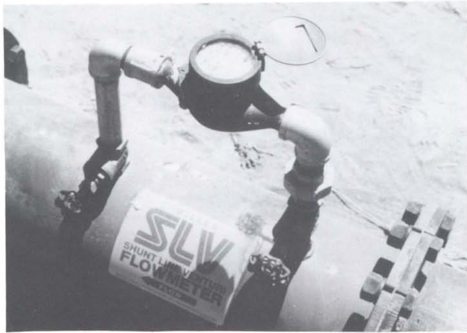
Figure 5. Miller SLV Shunt Type Flow Meter
