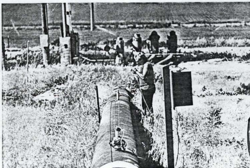
Figure 4. Triangle Dairy Pumping Station
