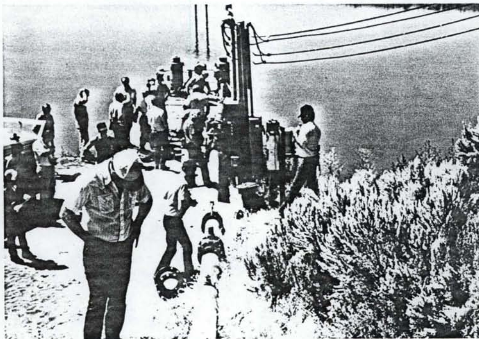
Figure 3. Ed Potucek Pumping Station
