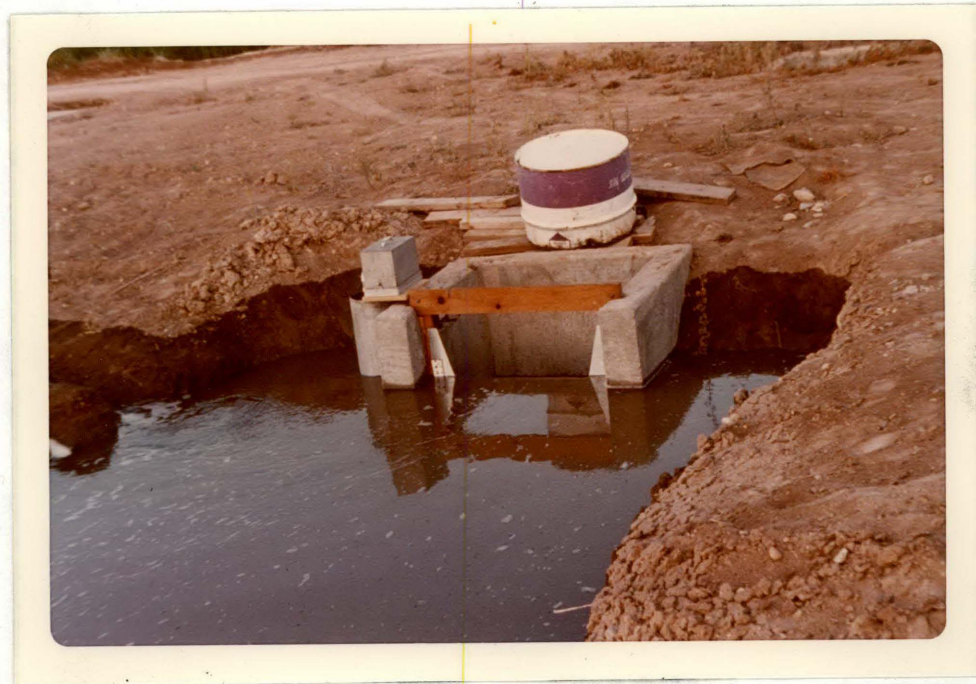
B. Structure after the two-foot adjustable cipolletti weir was installed
