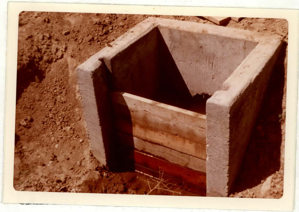
A. Structure at the beginning of the season before the weir and recorder were installed
