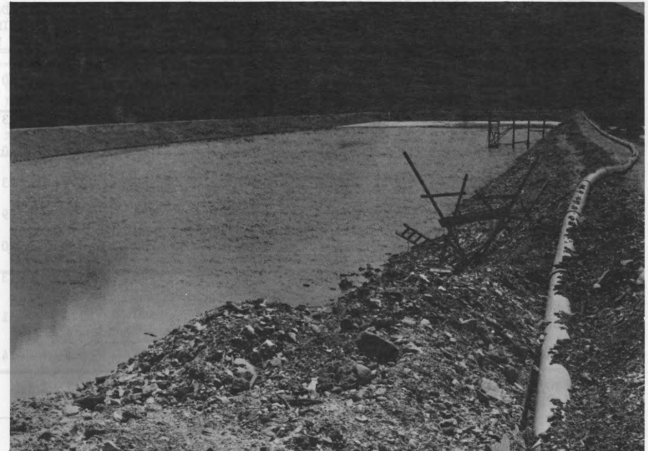
Slimes are now collected and stored in tailings impoundments.
