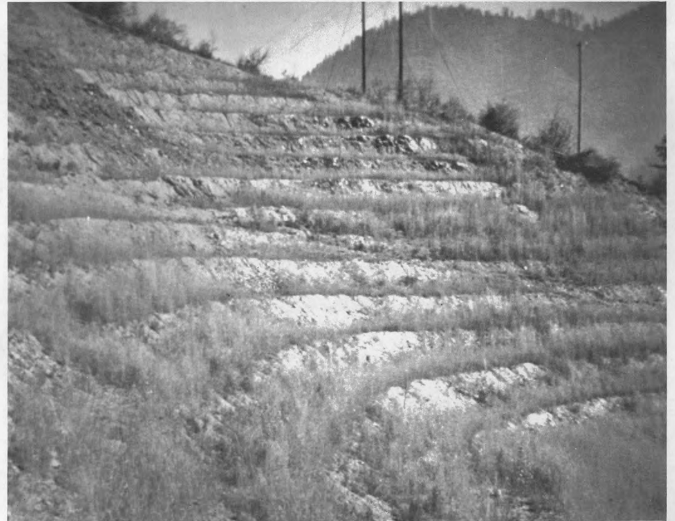
Serrated slopes help reestablish vegetation on highway cuts.
