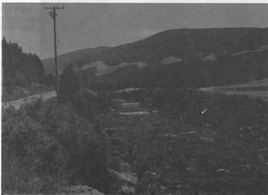
Construction of Interstate 90 above Mullan left scars on the hillsides as shown on the upper half of this photo.
