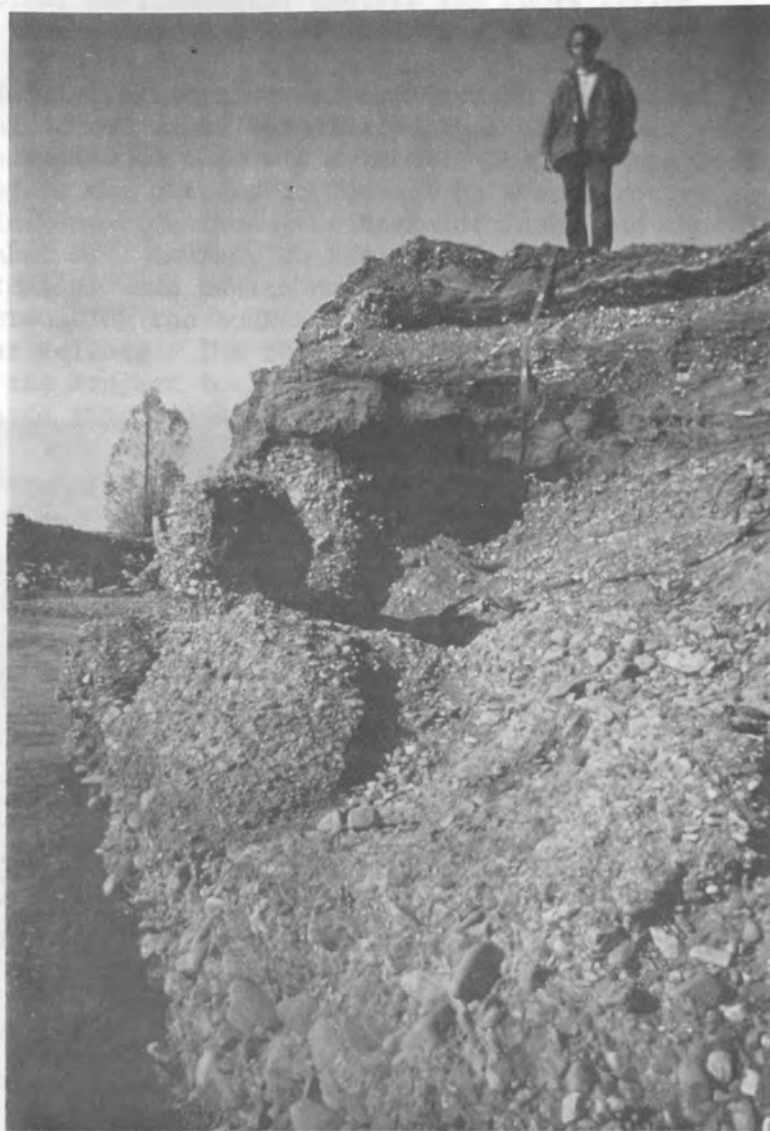
Stream bank erosion is prevalent along stretches of the South Fork.
