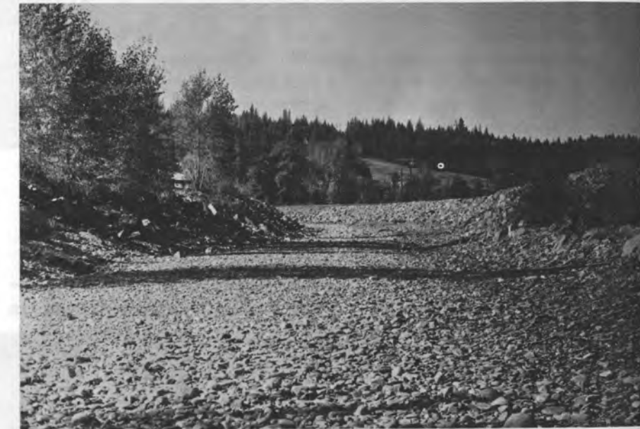
The 100-year flood channel on Pine Creek is not designed for fish habitat.
