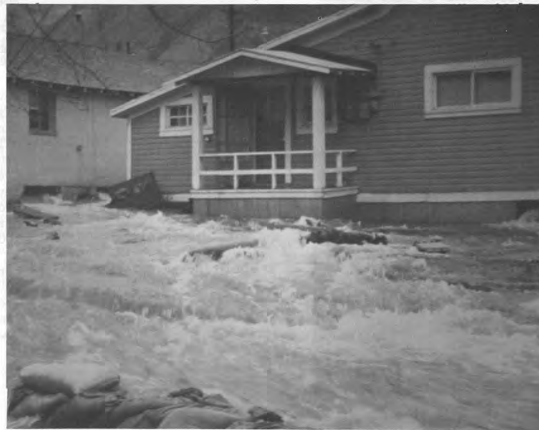
Flood damage was extensive during the 1974 flood.
