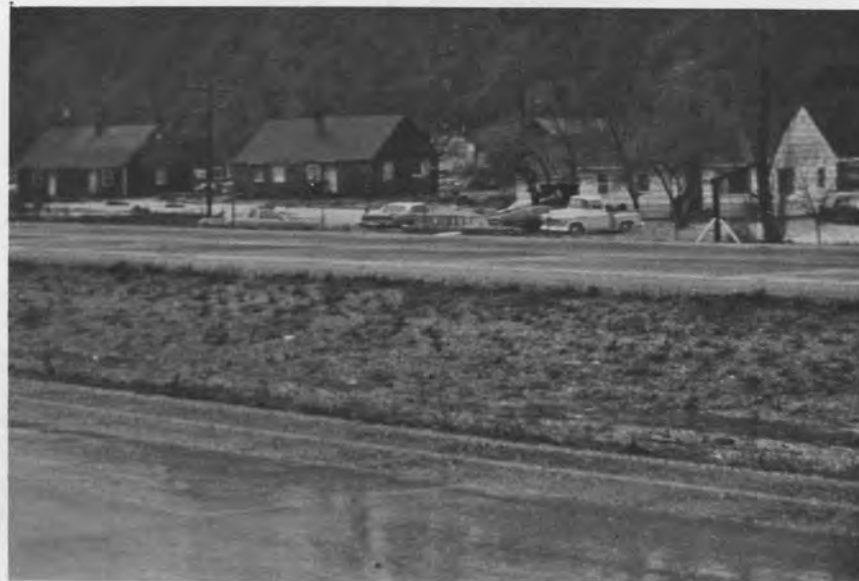
Flood damage during the 1974 flood.
