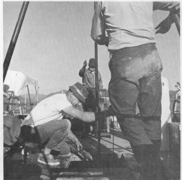
Figure 17. Lowering of Coring Mechanism until Trigger Mechanism Activates Free Fall.
