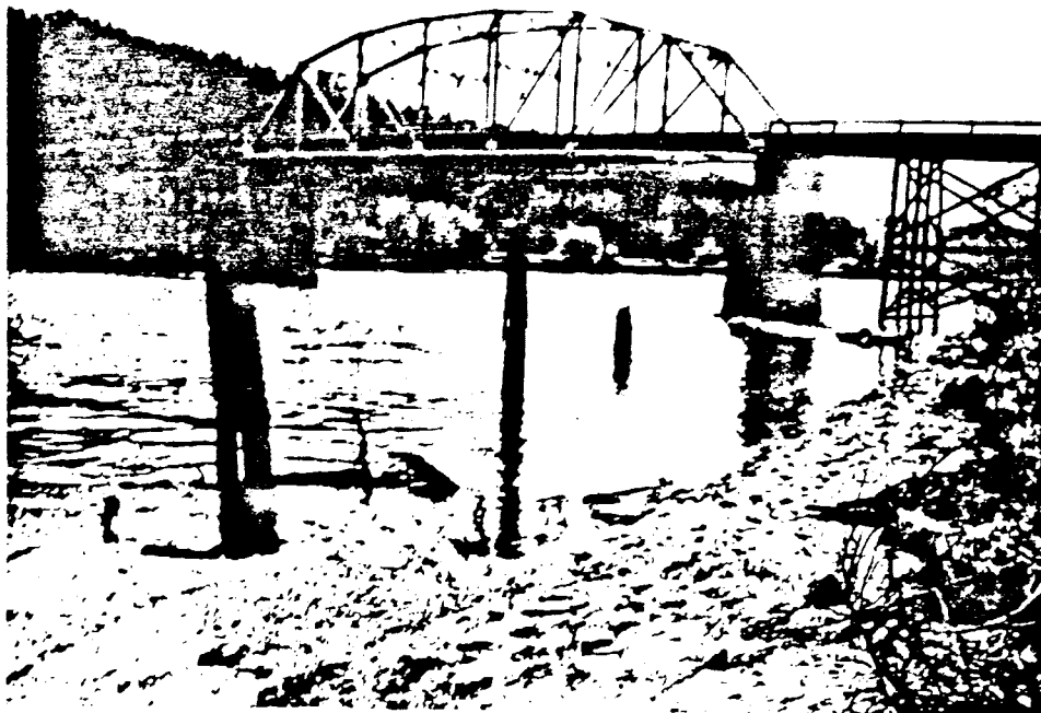
Figure B-14. State Highway 97 bridge near the mouth of the Coeur d'Alene River.
