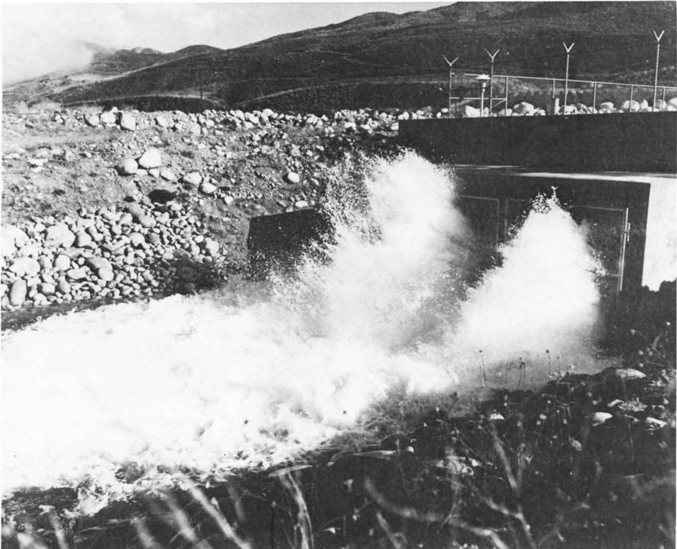
Figure 23. Waterman Outlet turnout — San Bernardino Municipal Water District.
