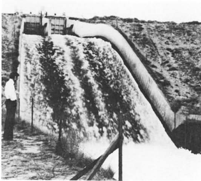
Figure 22. Check 22.7 Drop Structure — South Columbia Irrigation District.
