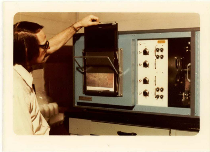
Figure 5. Additive color image combiner used to produce multitime imagery.
