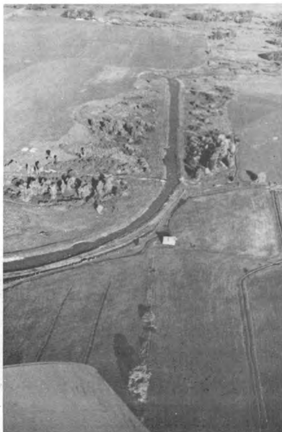
Figure 16. Channeling of the upper South Fork of the Teton River near Victor. The old channel meandered through the trees, but was straightened, resulting in increased water velocity.
