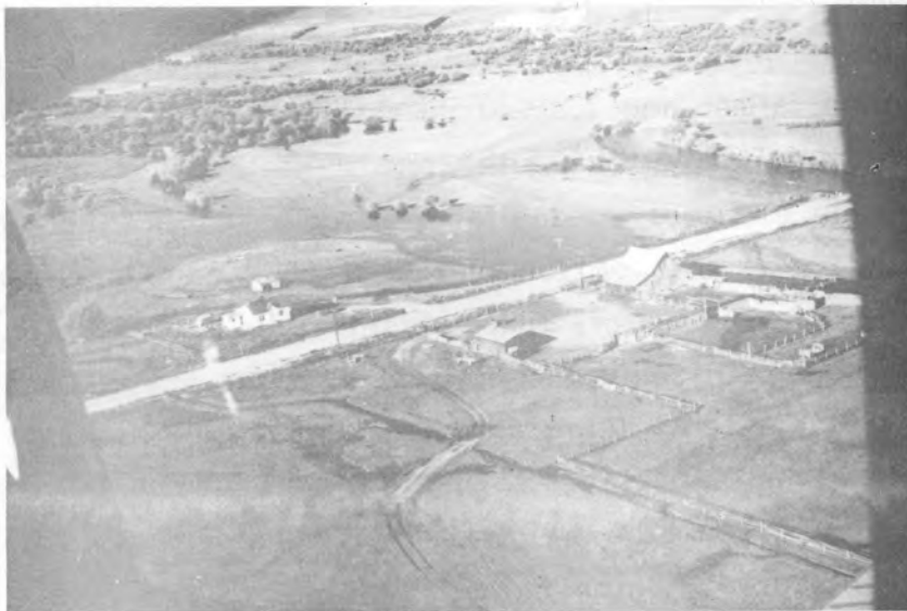
Figure 13. Flooding of the South Fork of the Teton River near Victor. Note the annual flooding problems that have occurred in the foreground. This is a normal spring flood which happens every year.
