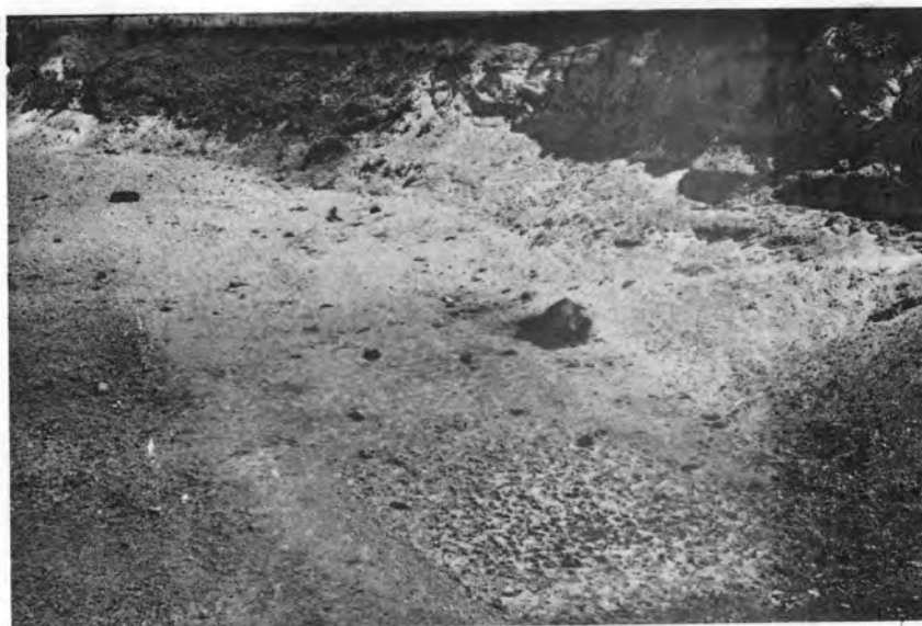
Figure 28. Additional accumulations of debris and dead cow in the eroded stream channel located on the Henry's Lake flats.
