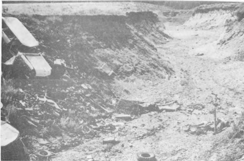
Figure 26. Badly eroded stream channels become receptacles for junk and debris dumped there by local residents.
