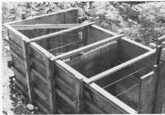
Figure 13. Tailbox of the 30.5 m culvert facility showing the upstream experimental compartment (right) from which test fish could ascend the culvert, and the downstream conditioning compartment (left) in which fish could recover overnight from any effects of netting
