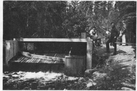
Figure 4. View of dam with inclined plane trap installed for the collection of downstream migrants (1974)
