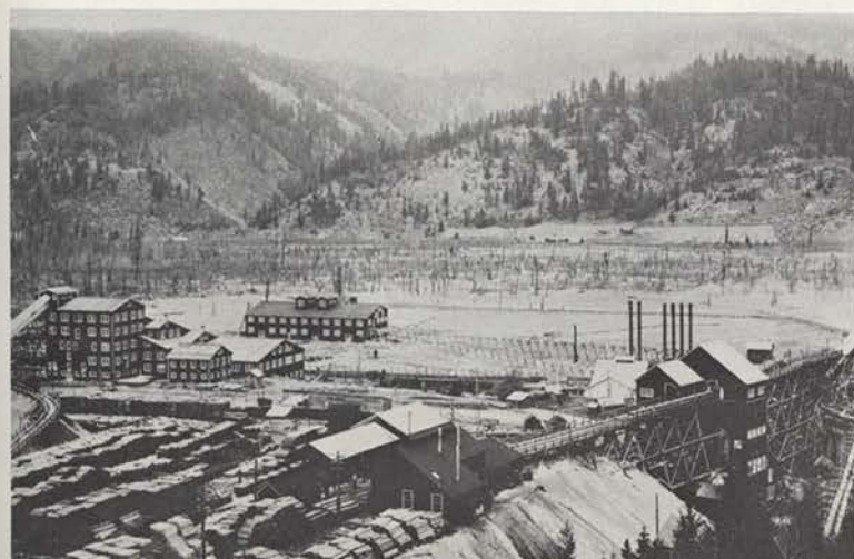
Mine tailings dumped in the river corridor at the turn of the century killed off many of the cottonwoods, conifers and other natural vegetation. Top: Bunker Hill and Sullivan Mill and river channel in 1904. Bottom: Same scene in 1909.
