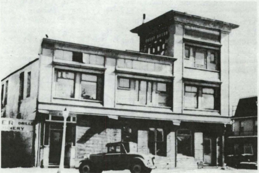
Above: Home near the university which Anthony designed and built for his family Below: Combined home and workshop on the northeast corner of Seventh and Main; Gritman Hospital at far right
