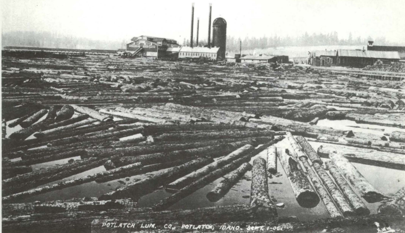
POTLATCH LUM. CO., POTLATCH, IDAHO, SEPT. 1-06. Mill and pond, September, 1906. LCHS collection.
