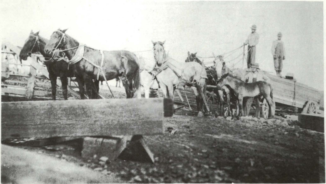
Hauling lumber for building construction, Deobald farm.
