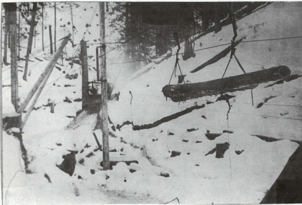
Highline Logging, with Donkey Engine
