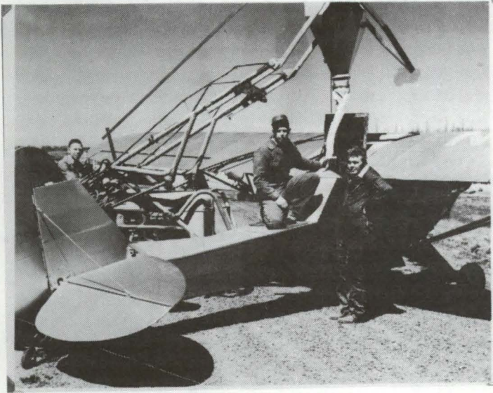
Filling the hopper of a converted Piper J-3. Pete Fountain on the right.
