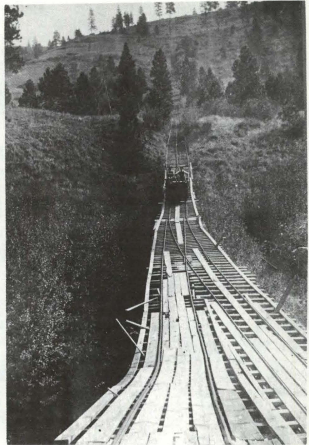
The Juliaetta tramway about 1912. As the cars approach the warehouse, the track divides so that they can be switched to the lower (right), or the upper level of the warehouse.
