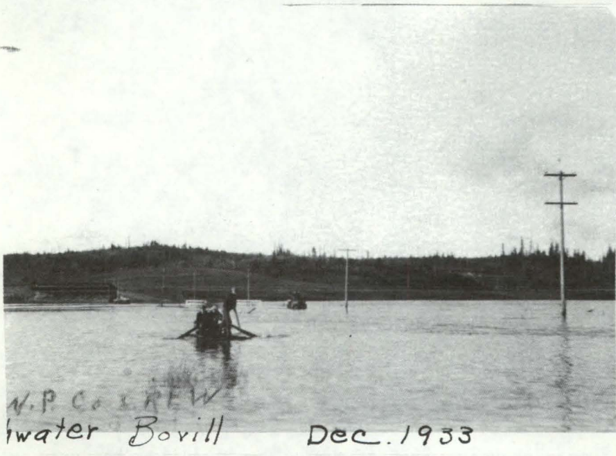
An infrequent hazard. Water over the creek banks and this WWP crew had to take to their boat.
