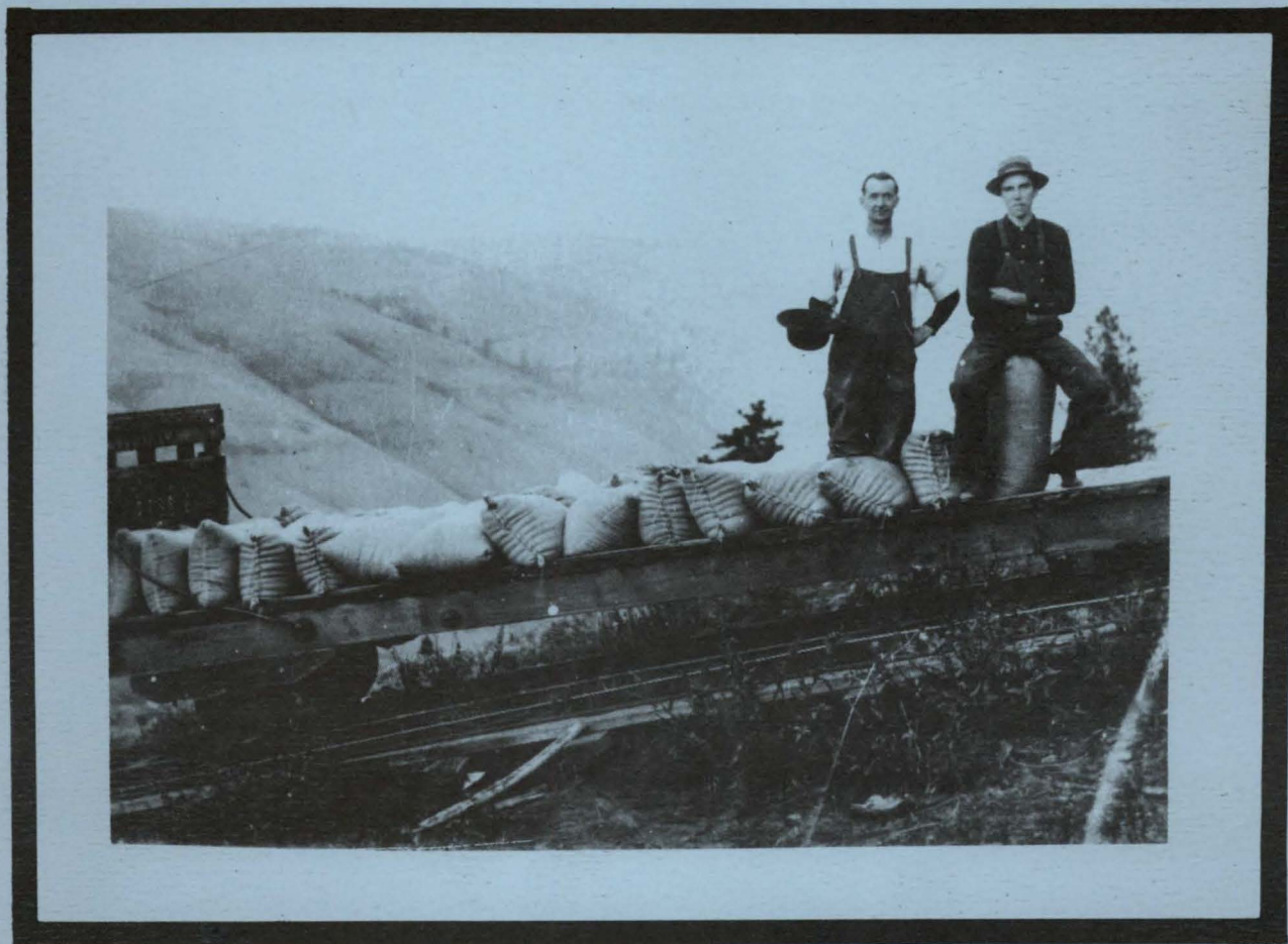
A tramway car partly loaded, and Arthur Perryman and Herman Schupfer at the top of the Juliaetta Tramway about 1912
