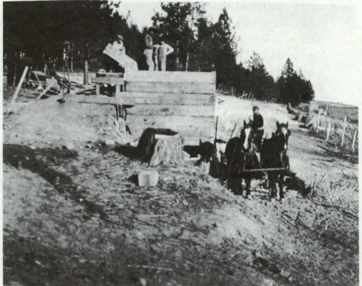
Building the new road near Viola, showing the rock crusher and gravel loaded into wagon.
