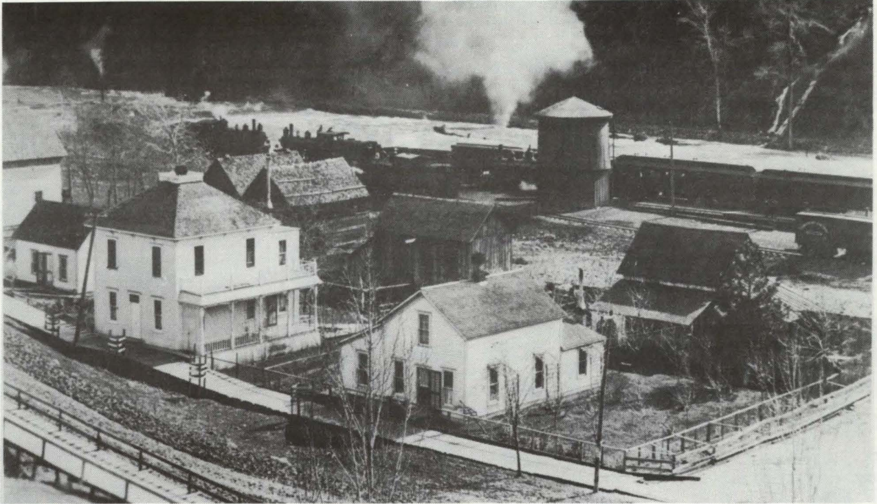
The Van Arsdol engineered railroad along the river bank in Kendrick. Note the high water which eventually led to the flood of 1900.
