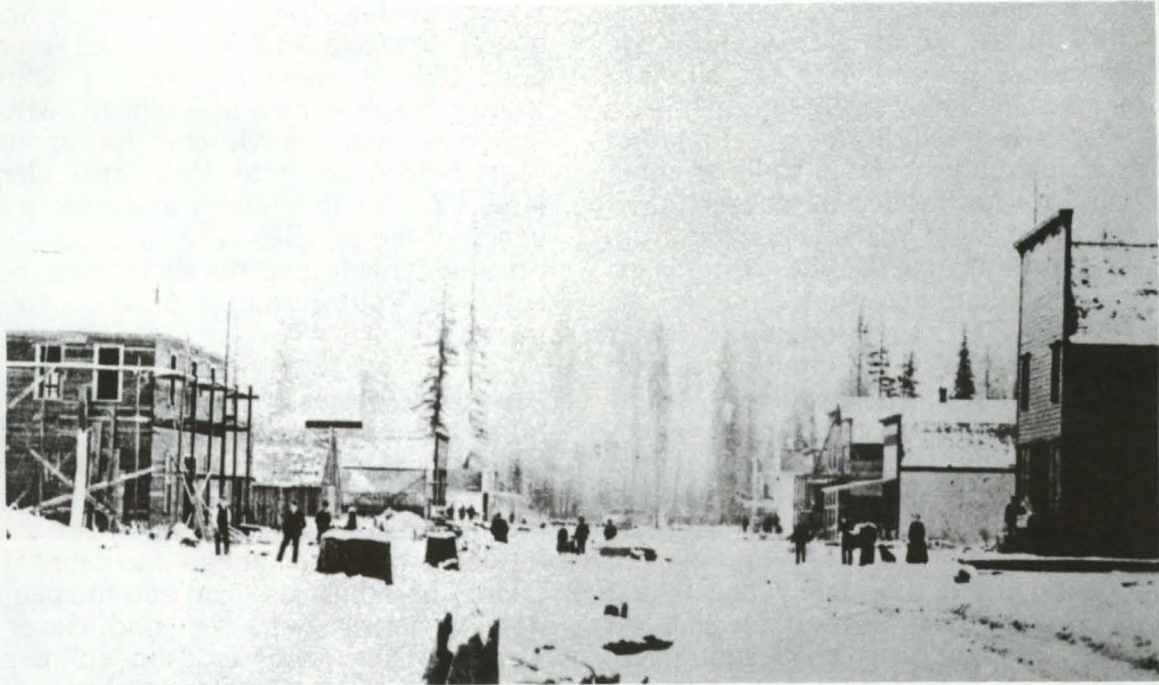
Buildings under construction in Vollmer in 1891
