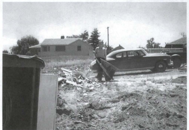
The individual in this photo is unidentified but could be Edward Moore. The roof of the addition to his house was blown off by a fierce gust of Palouse wind before he had a chance to secure it properly.
