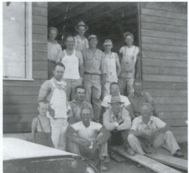
The gang's all here! The house-building professors take a break from their labor to have their picture taken in the doorway of what would soon be the house of the Malcolm Hause family. Bill Parish probably took this photo.
