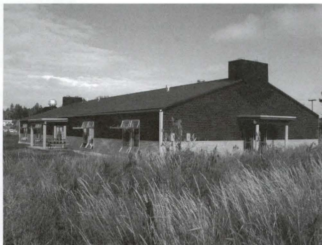
Building exterior, looking east.
