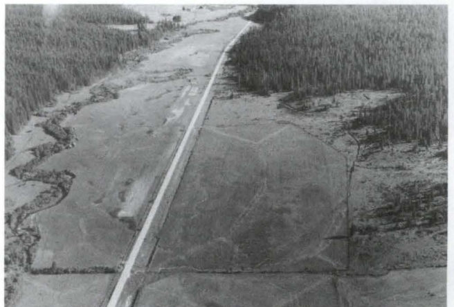
Aerial view of landing strip north of Laird Park along Highway 6.
