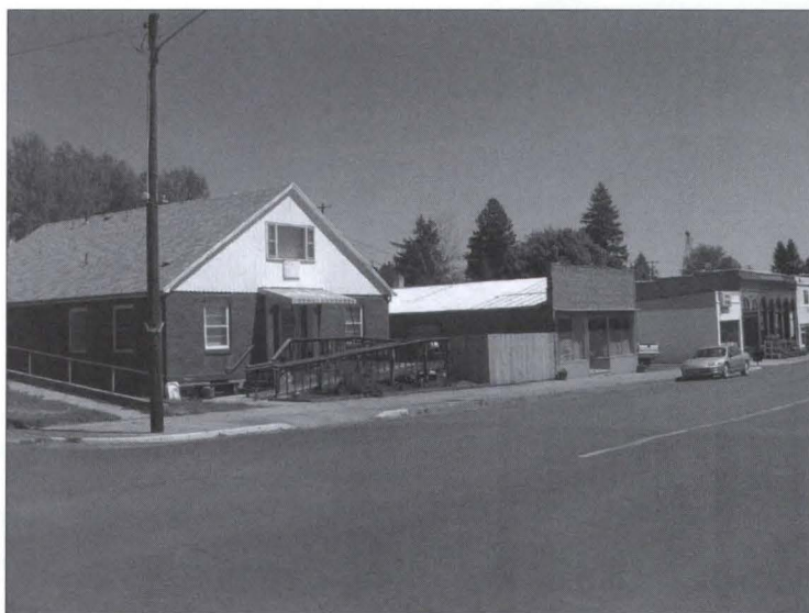
The Genesee Medical Center in 2006. The access ramp was built by Gritman when they operated their clinic in the building, courtesy of Earl Bennett
