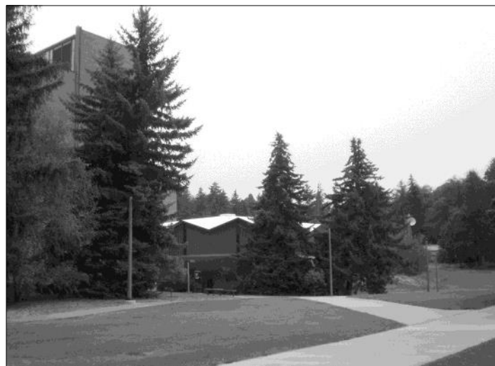
The Kiva lost in the landscape, facing southeast coming from the campus core, 2014. (Photo by Burns.)
