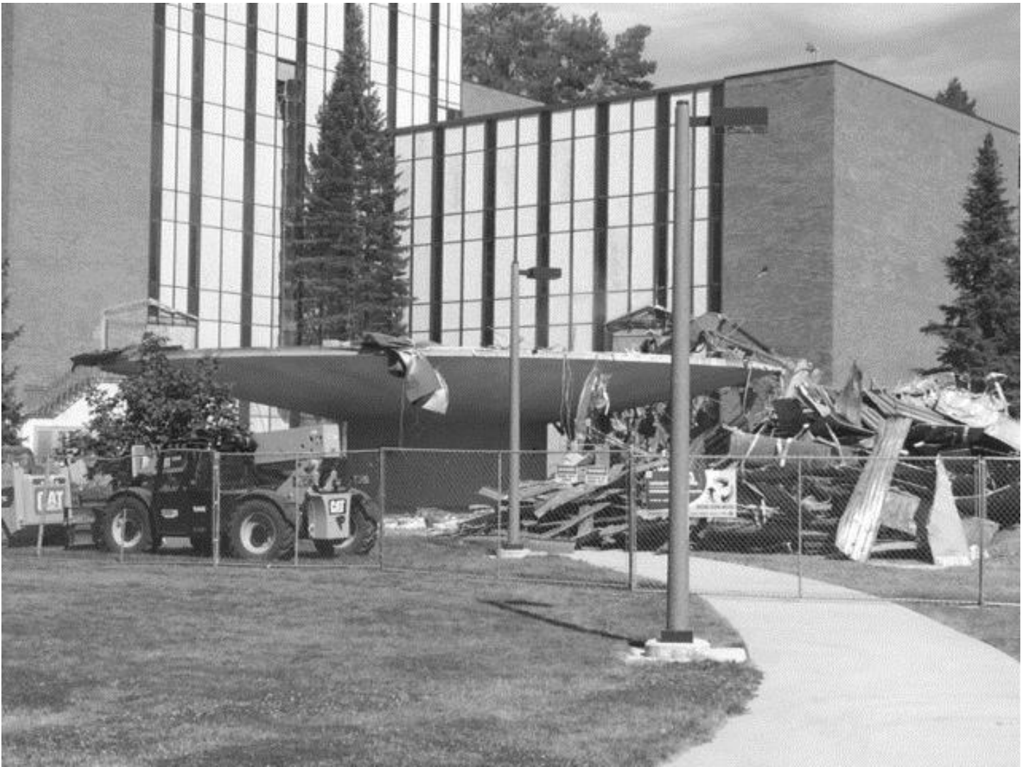
Kiva demolition, 2014. (Photo by Amber Ziegler.)
