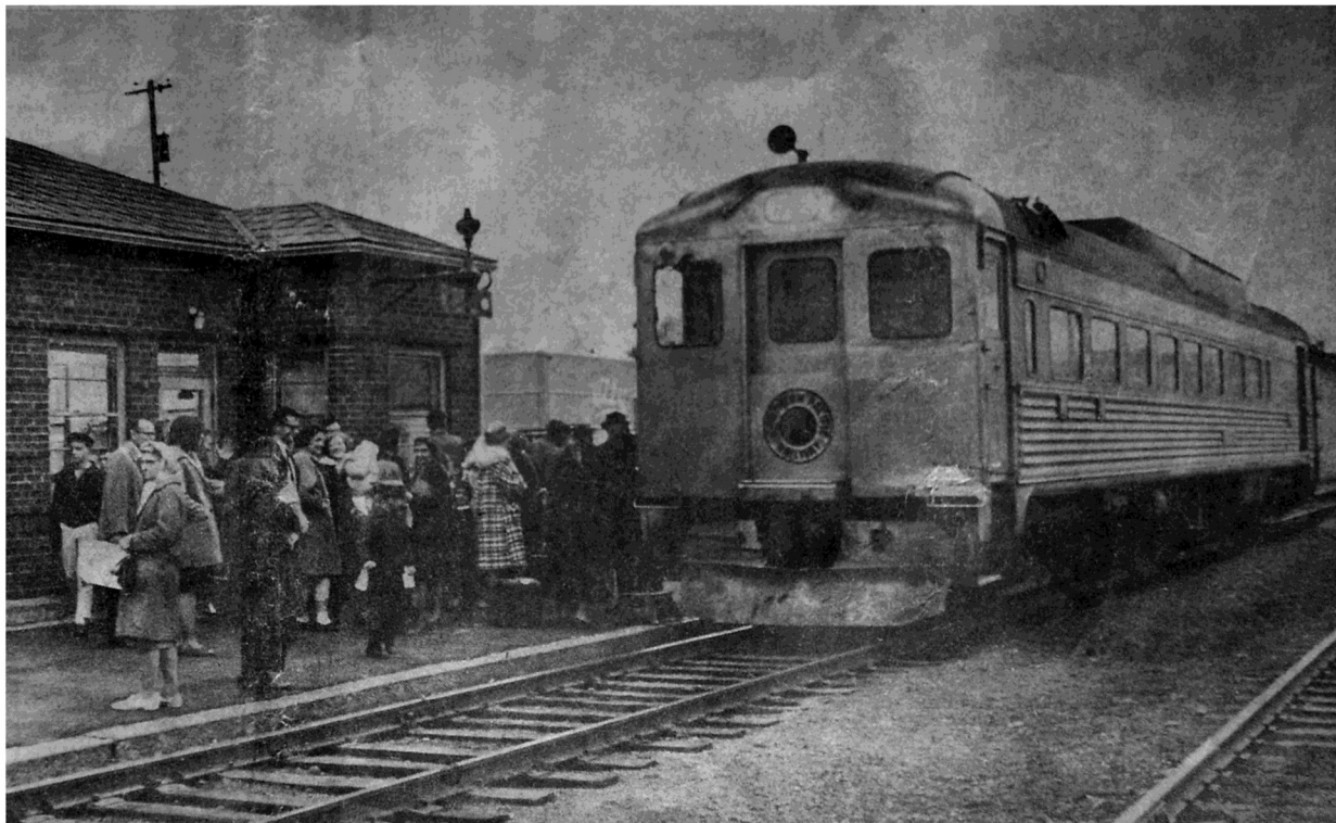
Figure 11. TOP: B12, on the left, was a gas-electric “Doodlebug” that served the Camas Prairie Railroad, both passengers and mail, until 1955. B30, on the right, was a rail diesel built by the Budd Company in 1951. (James M. Fredrickson photo collection) BOTTOM: B30 made its last Lewiston-Moscow-Spokane run in 1966. A total of 131 passengers boarded the train at Lewiston although the car’s capacity was only 96. The picture illustrates the public’s interest in the last train ride in Moscow. ( Lewiston Morning Tribune , March 6, 1966)
