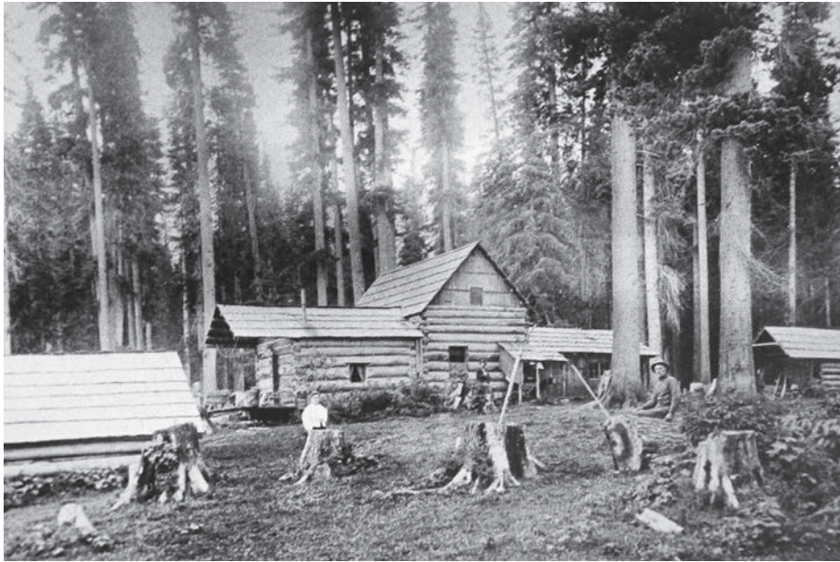
Homestead cabin near Collins (LCHS 03-05-001)
