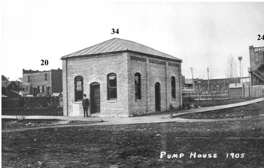
The Pump House at Chestnut Street and Laurel Street: 20. Alexander Building, 24. Conant Building, 34. Pump House. 1905. Clifford Ott Collection
